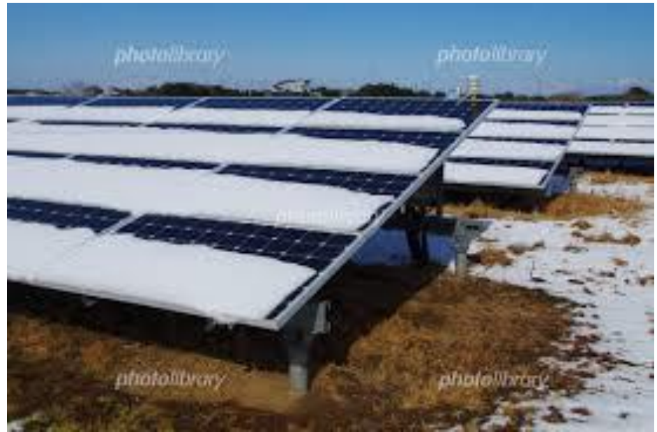
Flat solar cell during snowfall (does not generate electricity)
